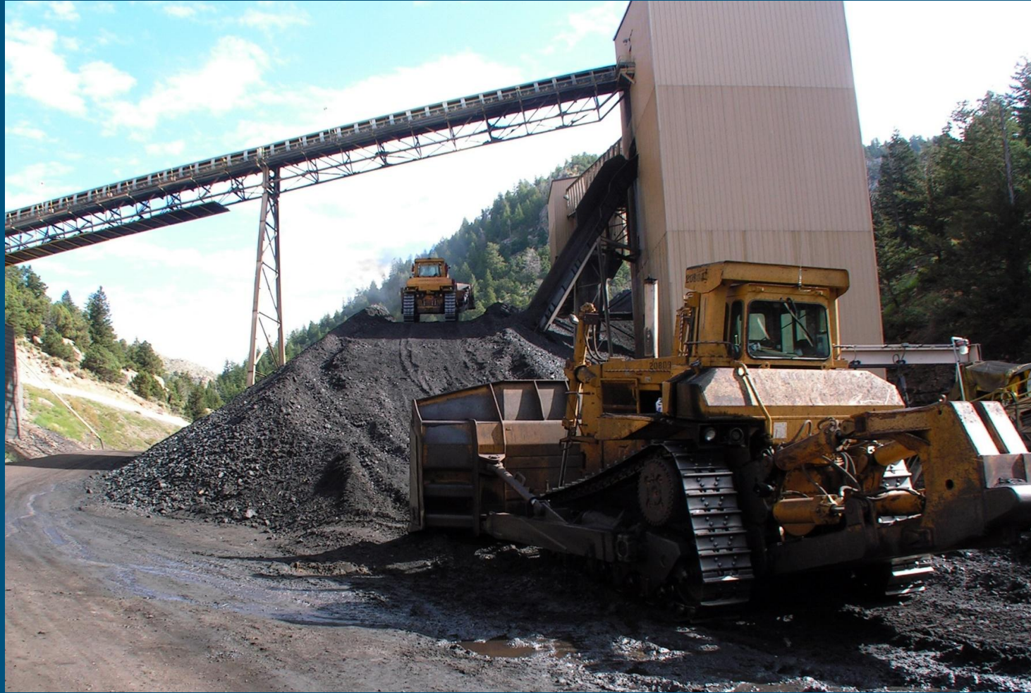
Coal Loader and Feeder – Carbon County
