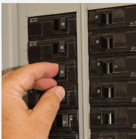
Locate the correct energy isolating device
